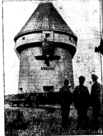
IT LOOKS LIKE A SILO —But underground 'are' de-scribing. It's a tower of reinforced concrete, along Germany's Siegfried line on her western frontier, designed to give shelter to 2,000 people. Nazi military spokesmen say it's "invincible." They contend it will withstand any attack from the air. The tower bears the name of a German World War flyer, Boelcke.
