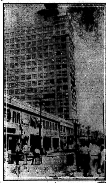
The Meyer-Kiser building, Miami, after the storm.
