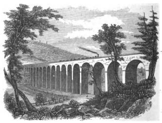
spans of 50 feet. Its body is 24 feet in width, but the top is 30 feet, affording space enough for a double track. Its appearance would be much improved by a parapet; but this deficiency is somewhat remedied by an iron railing on each side. Like the Cascade Bridge, the viaduct can not be seen to advantage unless you descend, and view it from various points below. The best of these is at the northeast angle, whence the beautifully-curved arches, and
