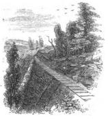
sage has made necessary. This is a heavy embankment, supported by a retaining wall 1000 feet in length and 30 feet high. We are now descending the slope of ten miles before us, and the scenery of the valley below is rapidly improving in interest and cultivation. A smile gradually breaks over the
