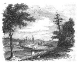
supported by arches of 160, 150, and 140 feet span, and rests on piers of solid masonry. Its cost was \$75,000.
