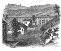
tion enabling us to look down the chimneys of that community. This tressle bridge is 450 feet long, and 70 feet above the Canewacta Creek, that here issues from a narrow glen, and is also a tributary to
